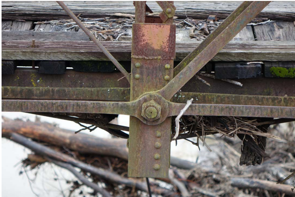
Photo 11 Bottom chord connection
